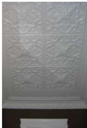
*Generally, the smaller the room, the smaller the repeating pattern. That said, a 24" pattern when combined with a filler panel and cornice can create a very dramatic effect.*
